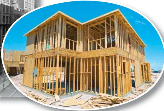
The frames went up quickly and provided both safe and strong dwellings. Almost all modern houses are still built this way. Even **skyscrapers** can be built with a type of stick construction that uses steel.
